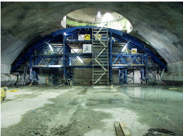
Figure 2: Vault concreting of ATLAS experimental cavern
