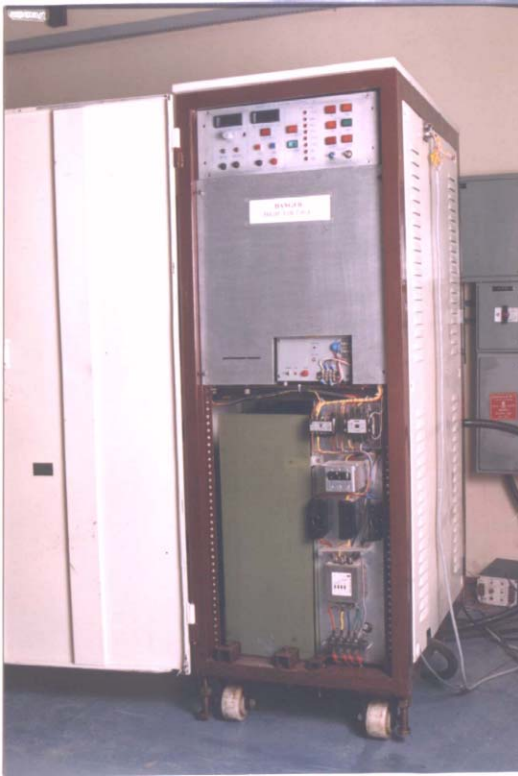
Figure 2: See From left Magnetron pulse modulator
