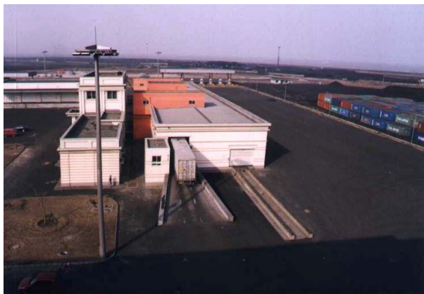
Figure 11: building and working field for the inspection system at the Tianjin seaport customs
